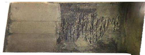
Figure 9. Orthoimage of the underside of the main deck of the unnamed bridge
